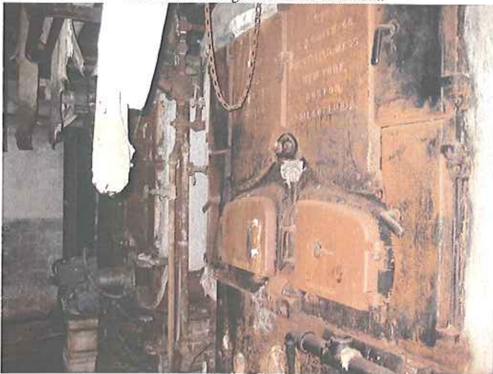
View of the boiler room.
