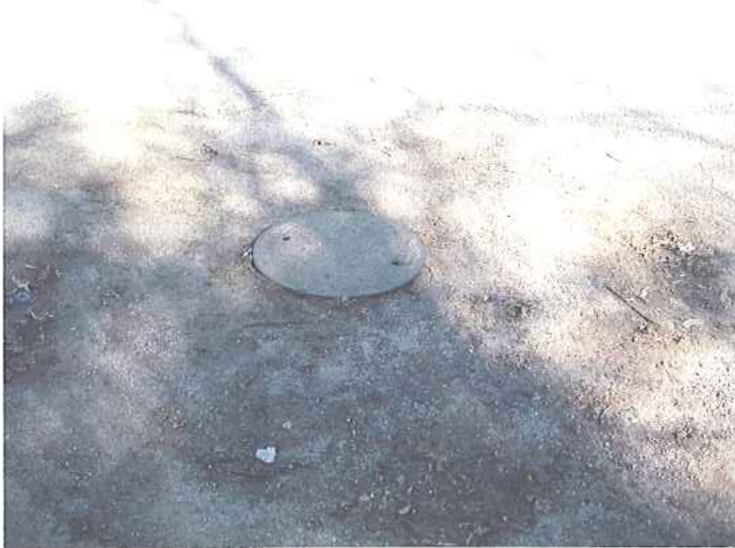
View of the solid cover manhole on the subject property.
